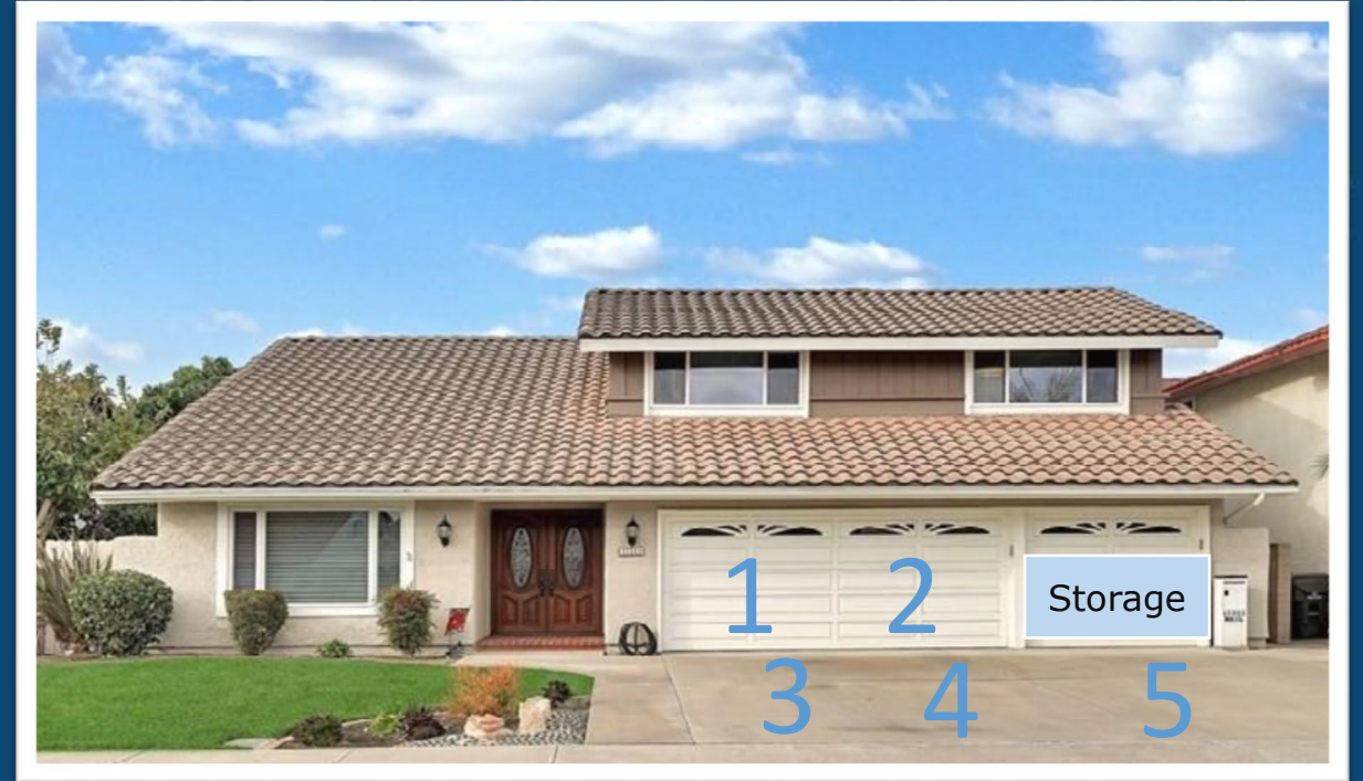
Three (3) car garage residence
